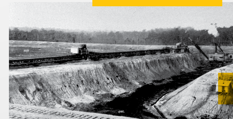
150B Bucyrus digging 600 ft trench through overburden to expose the first of Yallourn coal.
