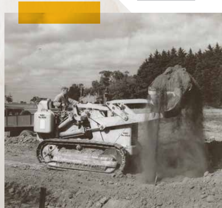
Allan Beech operating a No.933 Traxcavator on April 28, 1959
